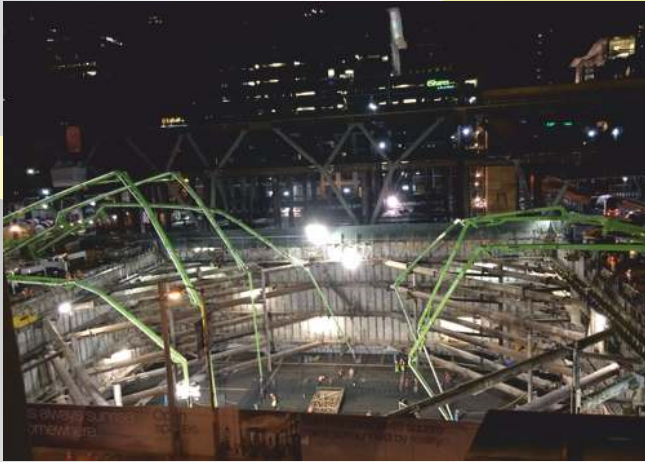
All seven Schwing CONCO booms can be seen discharging concrete early in the pour that began at 12:00 a.m. on a Sunday morning. Conco chose 4 Schwing S 58 SX and three S 47 SX concrete pumps for the marathon pour.
