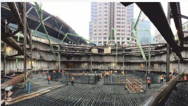
Six million pounds of rebar up to 2.25-inch diameter created a 14-foot mat to reinforce the concrete monolith.
