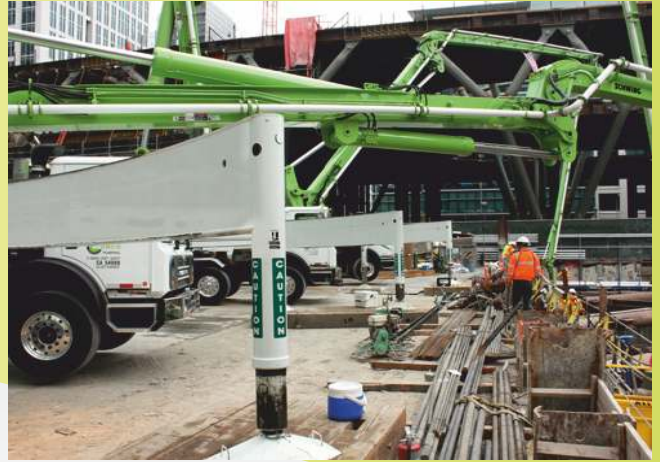
Schwing's exclusive Super X curved, telescoping front outriggers allowed seven of the long booms to fit on two sides of the excavation.
