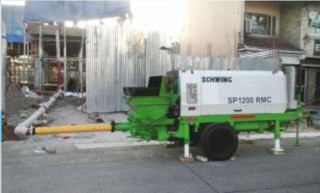
SP 1200 Concrete pump in operation
