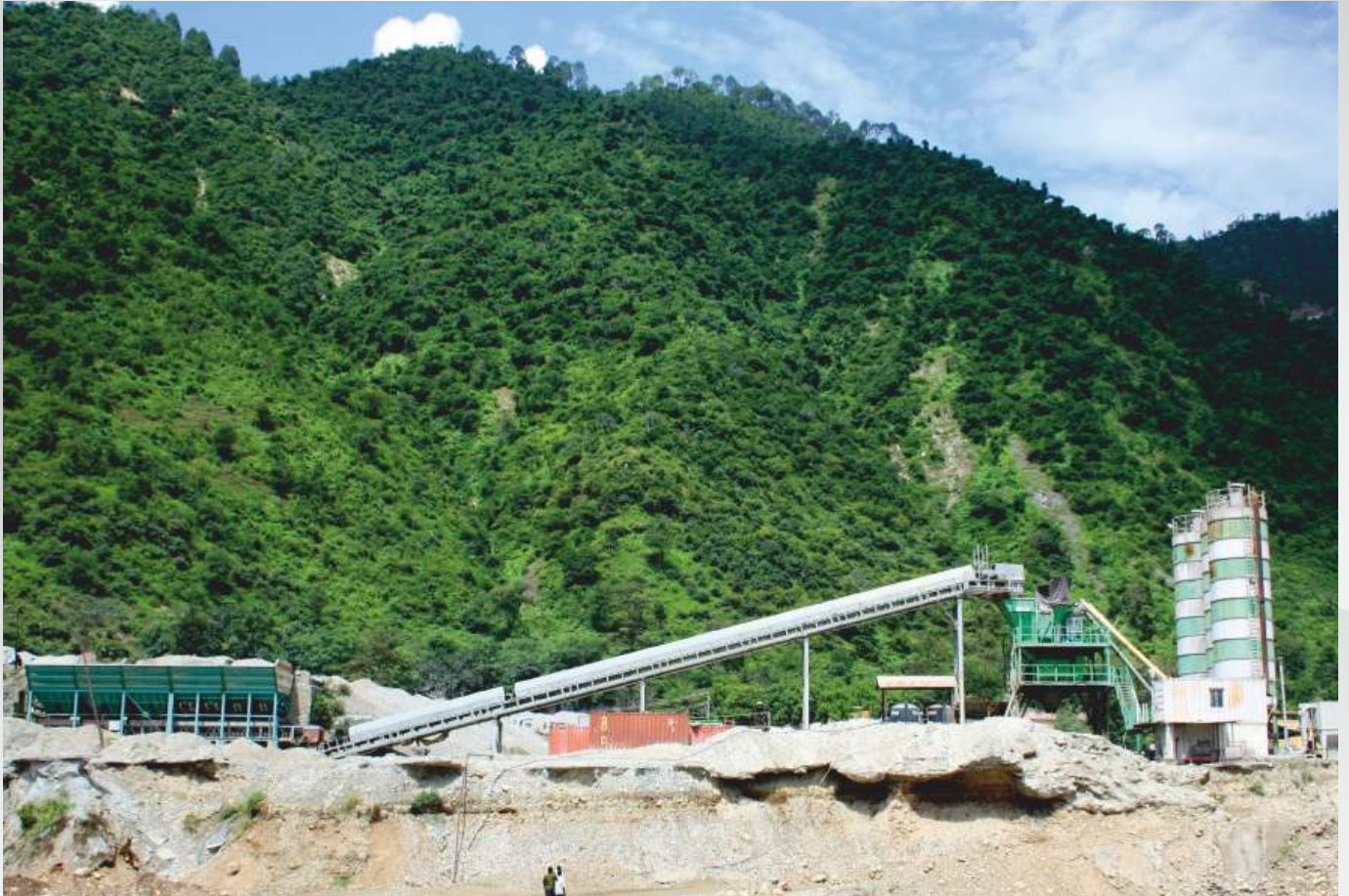
H4N 124 plant produced 6 lakh m 3 concrete also produced 35,000 m 3 in a month
