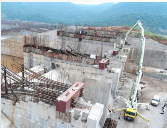
RET Irrigation project, Bhawanipatna, Odisha
