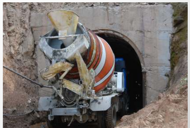
3 m 3 Nimo concrete mixer at tunnel concrete lining
