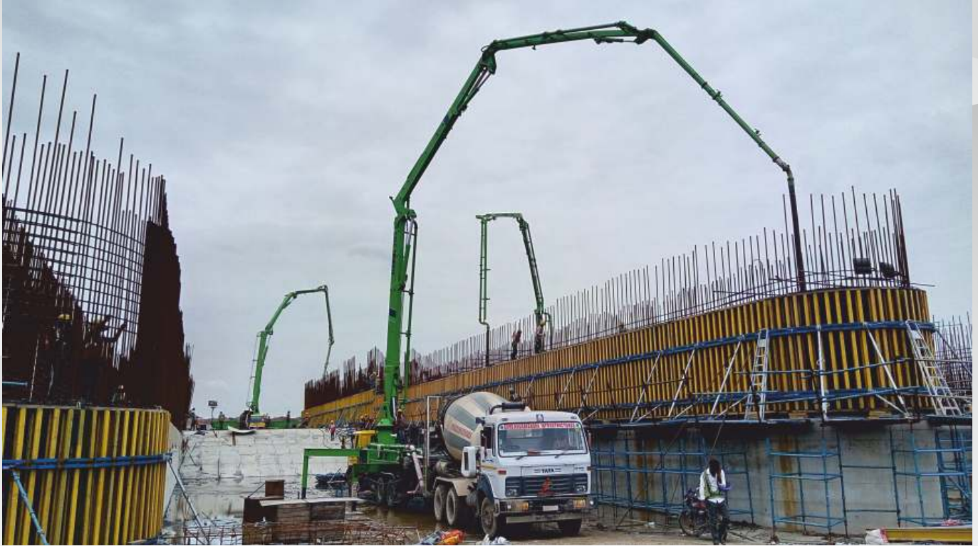
Kaleshwaram Lift Irrigation project
