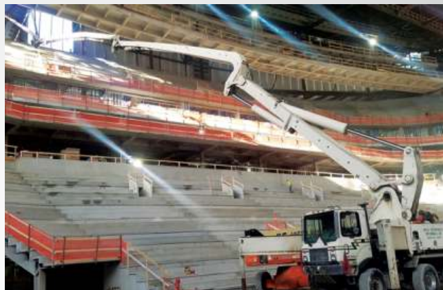
Schwing S 58 SX Long booms contributed to the efficiency of concrete pumping
