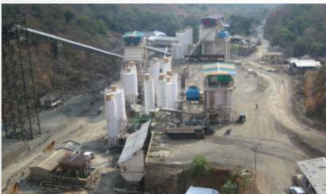
Ghatghar Roller Compacted Dam
