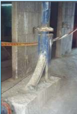
Long-radius riser bend secured in concrete.
